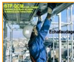
Echafaudage 2007 OPCA AREF Ile de France - Paris
